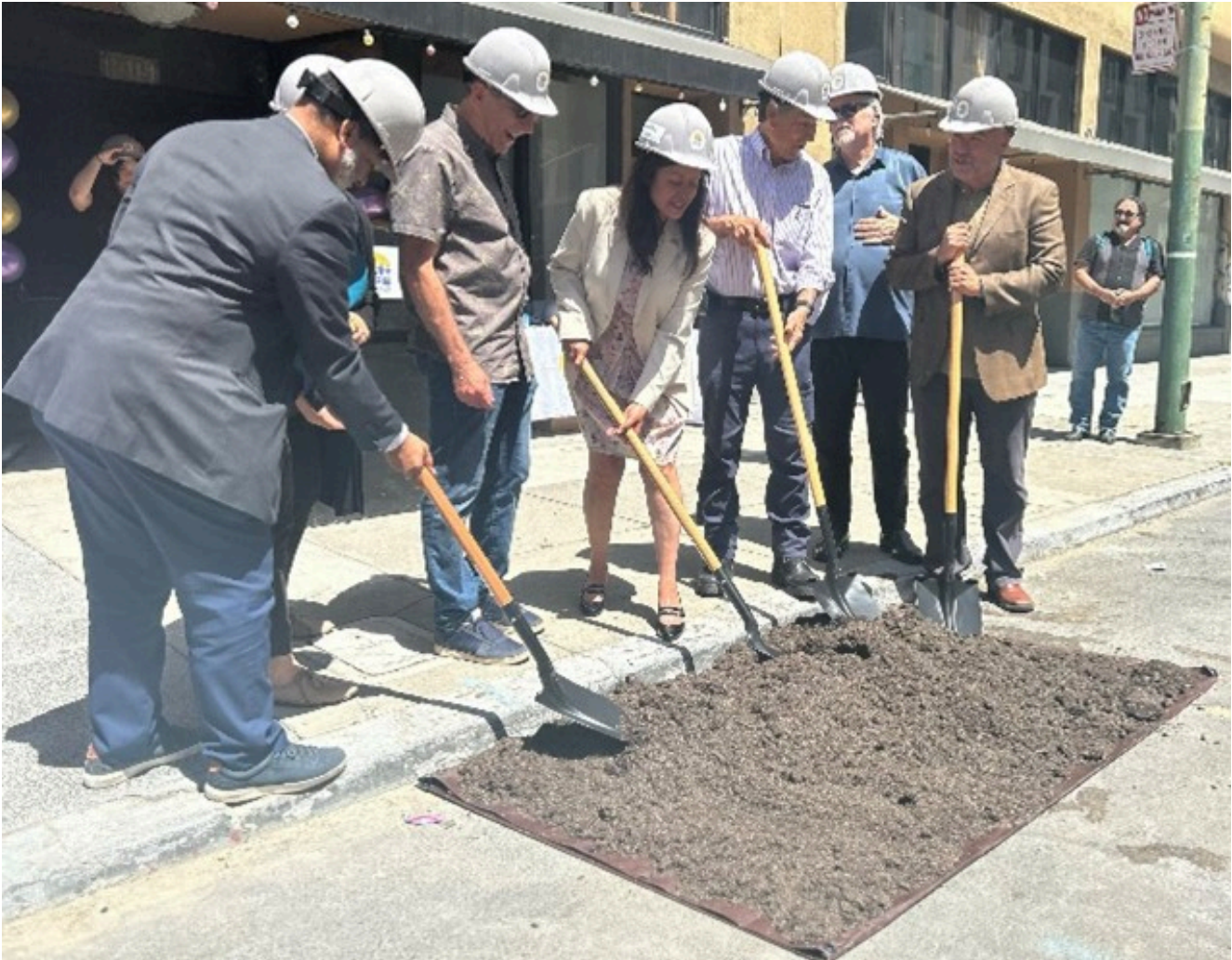
Groundbreaking led by Safe Passages CEO Josefina Alvarado Mena-center.
